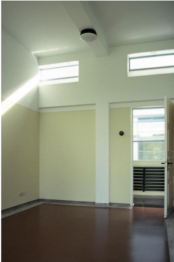
Sanatorium Zonnestraal, Hilversum (NL), archs. J. Duiker and B. Bijvoet, 1926-28, Main Building. Interior: bright light yellow walls with blue steel windows, brown linoleum in order to economize. Photo: Mariël Polman, 2003 ©Polman
